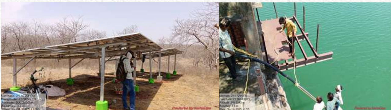
Image 5.6.3. Water management with installation of a 10 HP solar-powered pump at Karanpura in Gandhi Sagar Wildlife Sanctuary ©Madhya Pradesh Forest Department
